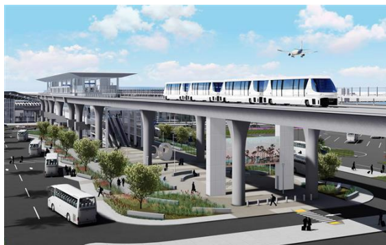
Figure 2. Example of Automated People Mover (Photo: LAWA)
