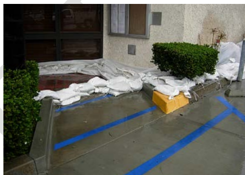
Water intrusion affected the emergency communications room at City Hall (located on the other side of this wall)
