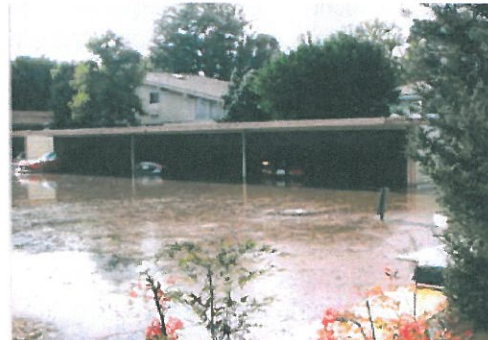
A carport in Laguna Woods Village cul-de-sac 67 flooded during the December 2010 storms
